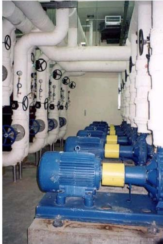
GHP equipment at Beijing Concordia International Apartment Building.
